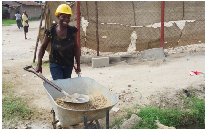
Figure 6: Local women were engaged during FSTP construction
