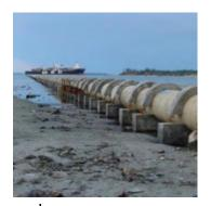
**Disposal / discharge outlet:** is the point where stormwater and treated wastewater is released back into the surface water bodies, e.g. ocean or rivers.
