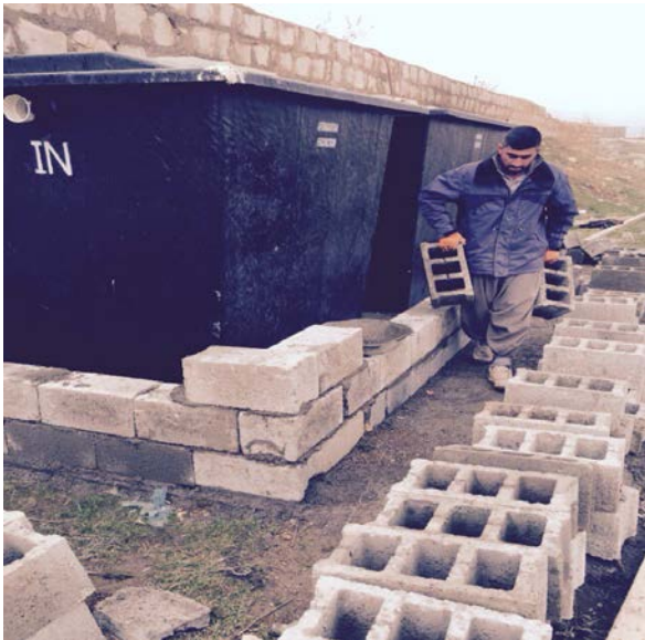
Figure 3: Construction of concrete block wall
