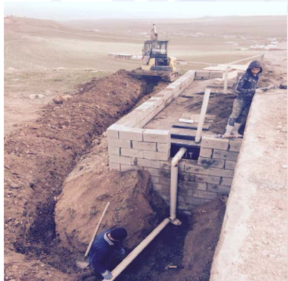
Figure 4: Installation of 4 inch outflow pipes
