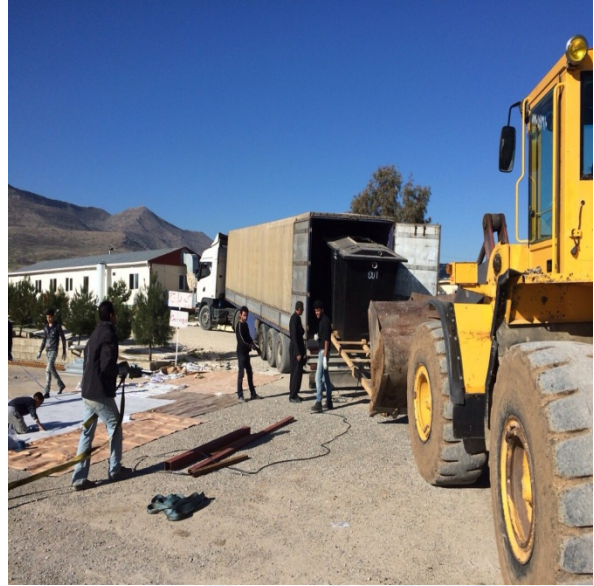
Figure 2: Unloading of prefabricated DEWATS
