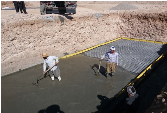
Figure 3: Reinforcement work and casting
