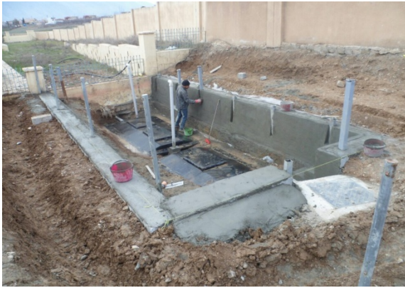
Figure 3: Low slope governs the installation of DEWATS 1.5m lower than natural ground level
