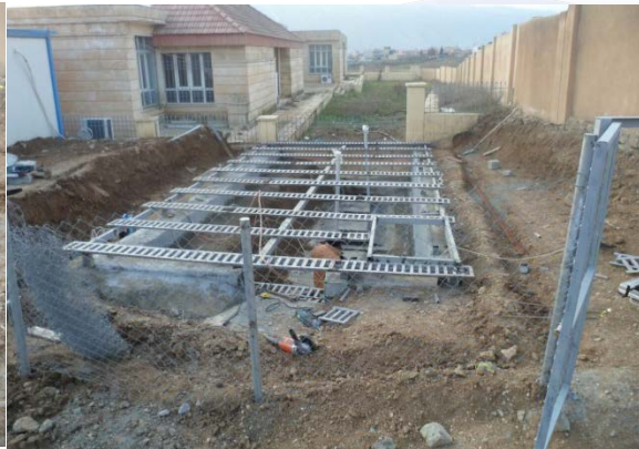
Figure 3: Low slope governs the installation of DEWATS 1.5m lower than natural ground level
