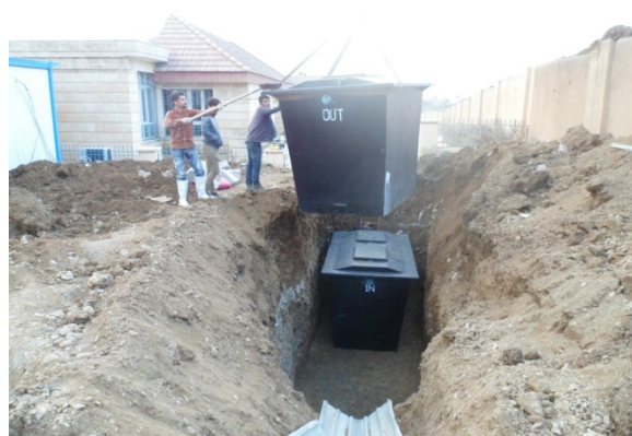
Figure 2: Casting concrete for foundation and installation of prefab-DEWATS
