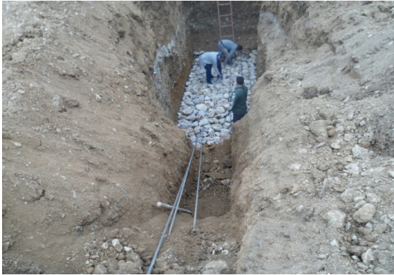
Figure 1: Excavation and crushed stone layer
