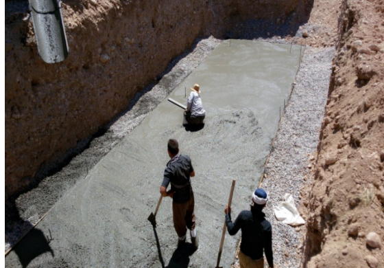
Figure 2: Laying 10 cm gravel layer and casting
