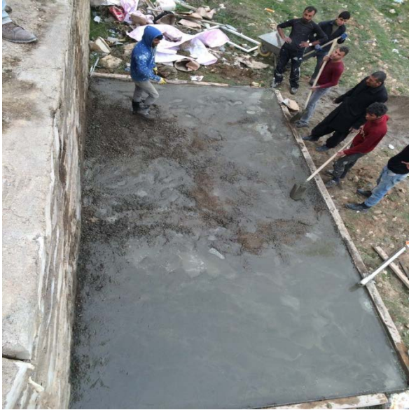
Figure 1: Casting of concrete foundation
