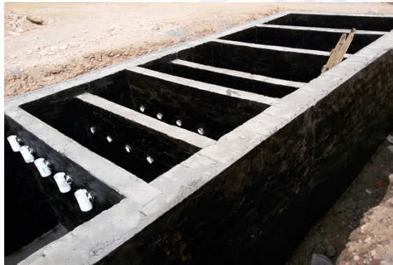
Figure 4: Finished wall covered by cement
