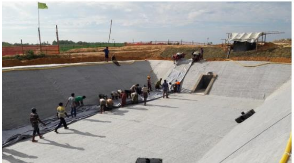
The sewage treatment plant under construction in Cox's Bazar
