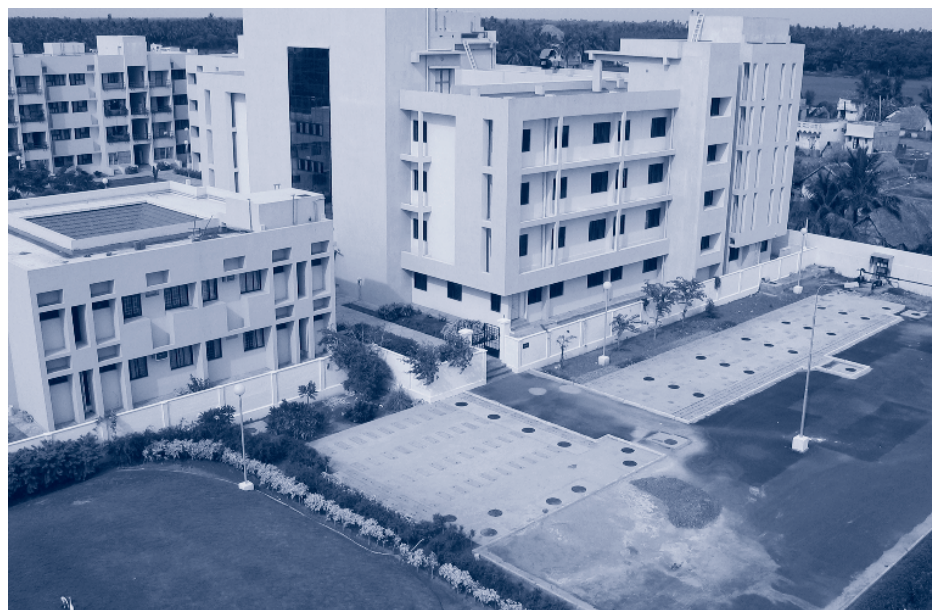
Picture 3_20: Baffled reactors are used as a parking lot
