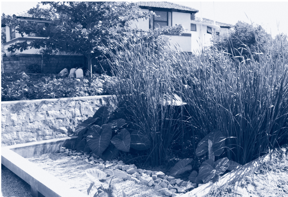
Picture 9_22 Horizontal gravel filter in India
