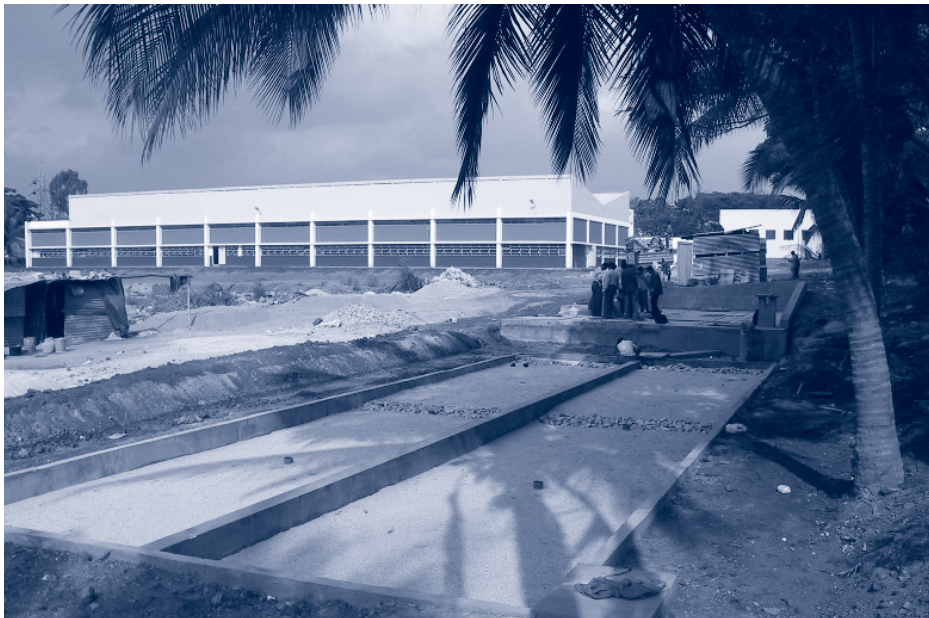
Picture 9_27: Horizontal Gravel Filter during construction. Constructed above ground
