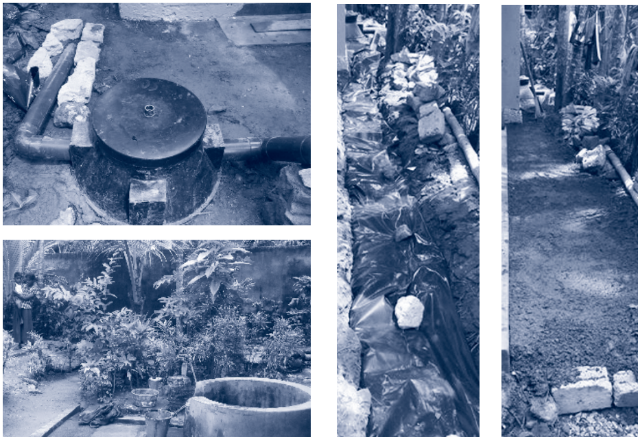
Picture 11_17 to 11_20: Construction of a French-drain filter, connecting a plastic septic tank with a plant-bed
