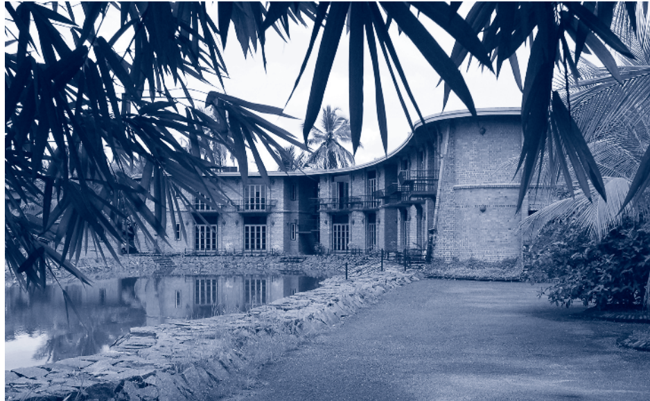
Picture 7_6: DEWATS at a Hotel in Cochin, India; large-size ponds are used for post- treatment
