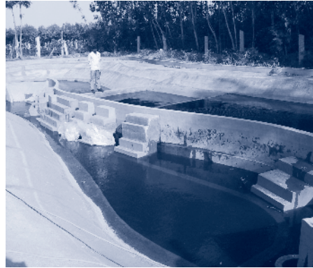
Picture 3_28: The anaerobic filter under construction
