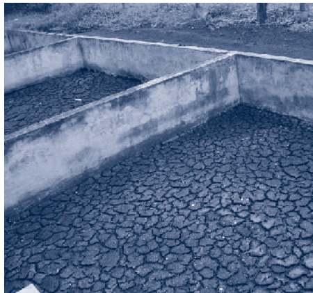
Picture 11_34: Sludge-drying bed and well-stabilised, small sludge cluster. Credit: A. Schmidt
