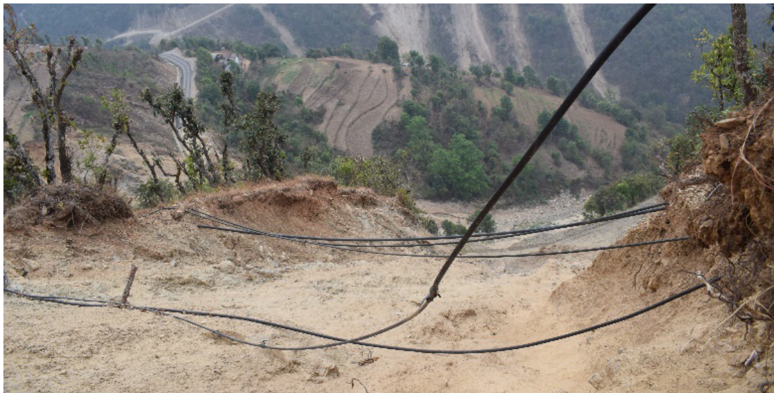
Figure 5: Landslide affecting the pipelines from water sources
