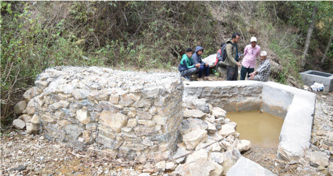
Figure 6: Contaminated intake
