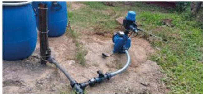
BORDA installed this portable booster pump to allow the drinking water to be supplied directly to the classroom to prevent kids having to walk during teaching hours to get drinking water.
